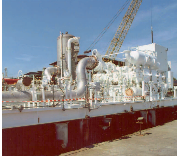
View of the compressor assembled on the skid
