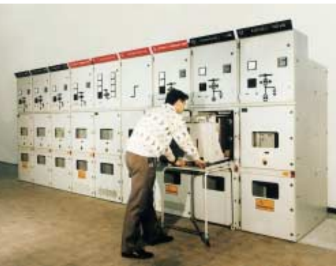
Air-insulated switchgear, type ZS1
