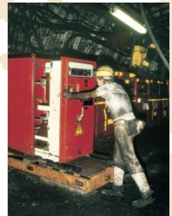
Flameproof switch panels, type ZE in underground mining
