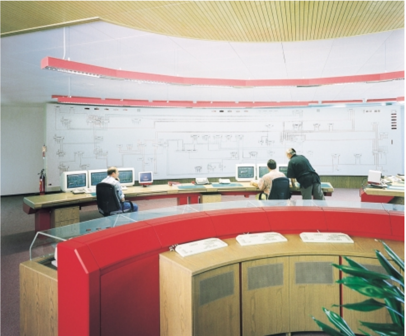
Operations control center in Mühleberg
