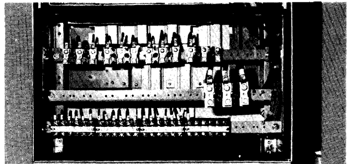
Figure 33. Typical Type C terminal board at bottom of section.
