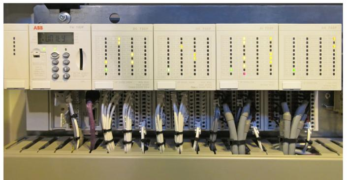
The Freelance controller AC 700F with S700 direct I/O
