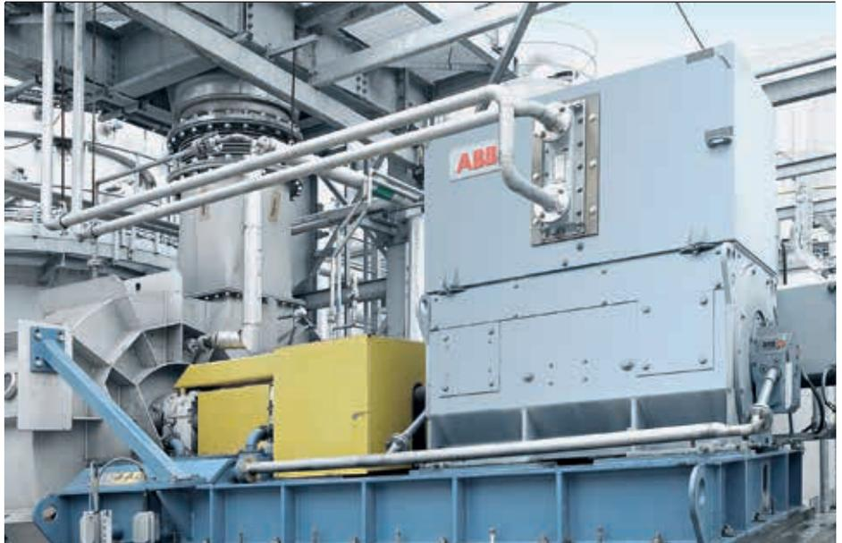
A typical power transmission chain consists of a driven machine – such as compressor or pump – an optional gearbox, a motor, an optional frequency converter and the power grid. These individual components are mechanically and electrically coupled and the power needed to perform the final useful work, such as accelerating fluid in a pump, flows through each of them. All the components must endure this power flow, which appears in mechanical components as torque.
