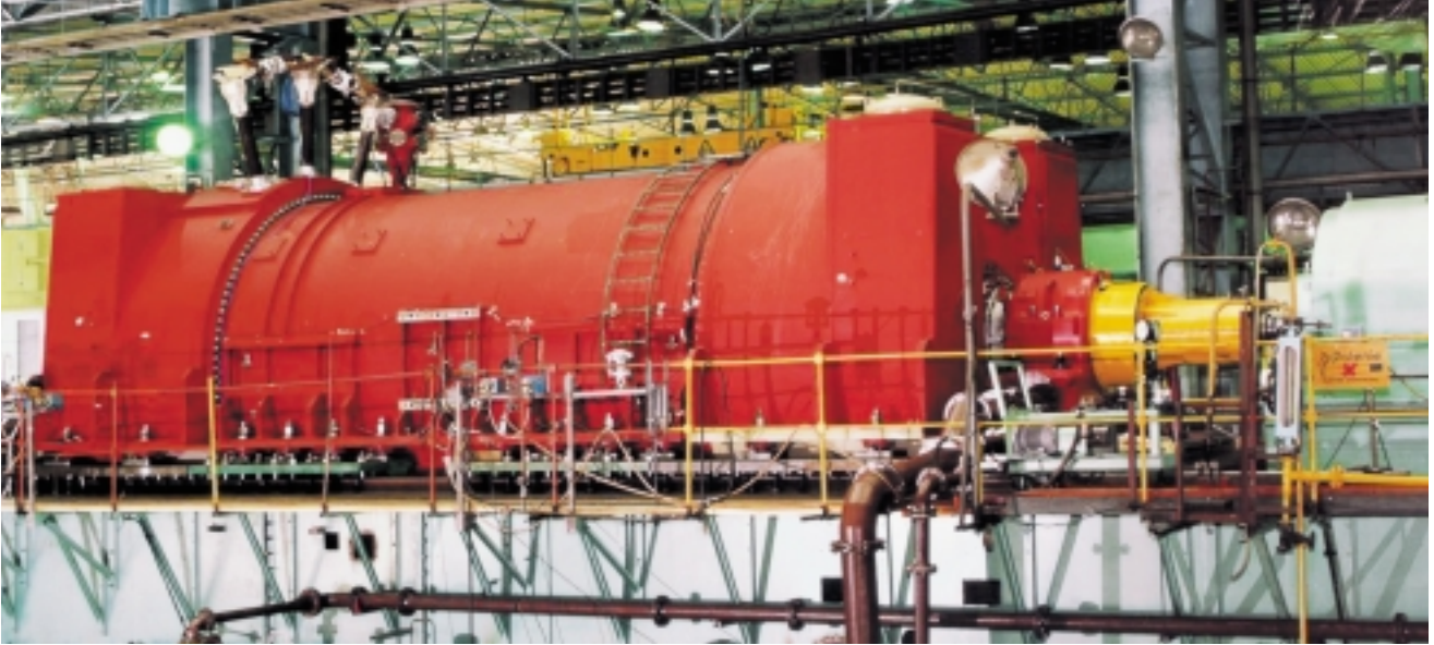
Indirect hydrogen-cooled 'Topgas' generator in the 500-MVA power class
