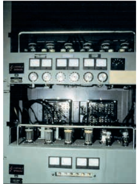
1 Original Gotland converter firing control system based on vacuum tubes
