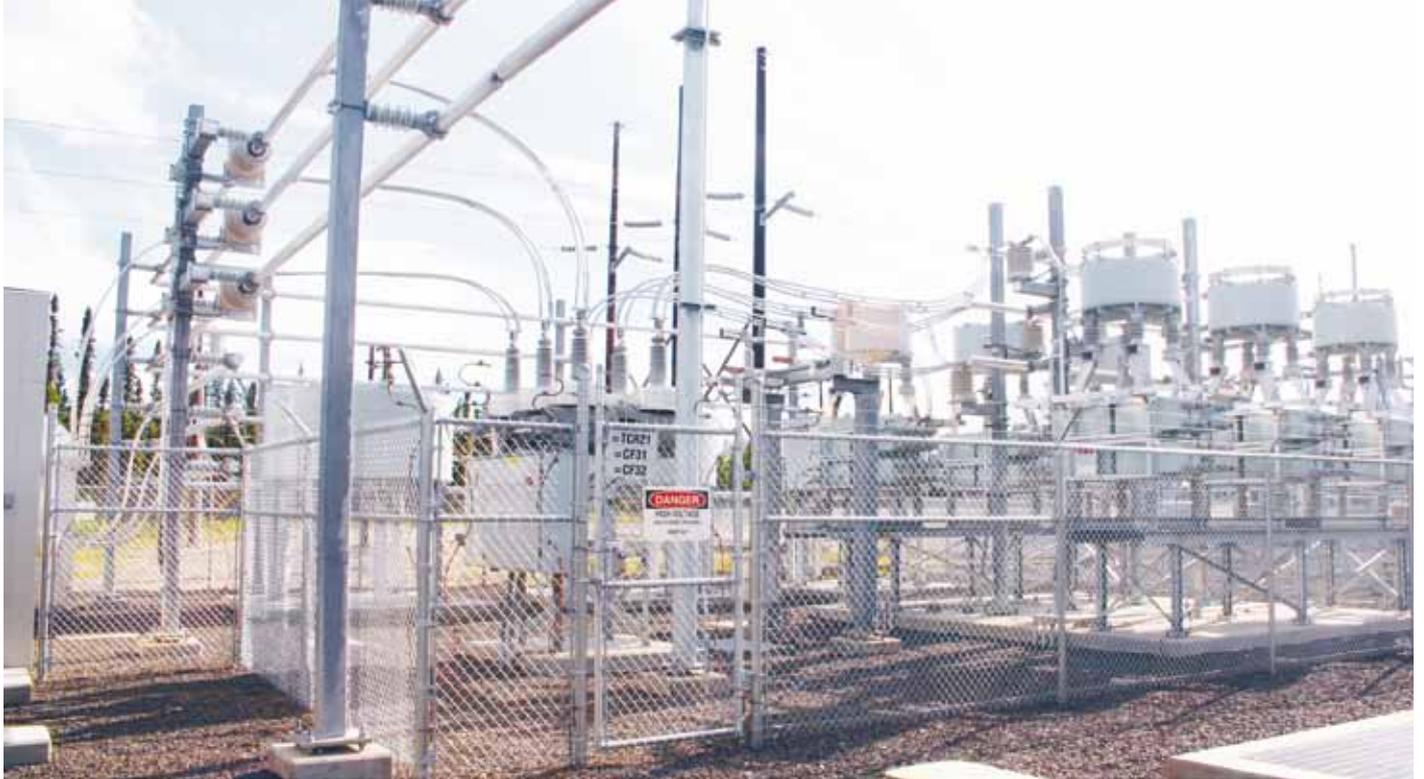
Golden Valley Electric Association (GVEA), located in Fairbanks, Alaska, is operating a Static Var Compensator (SVC) in their 138 kV grid, supplied by ABB in 2005 as a turnkey project. The SVC, located at Jarvis Creek in the Delta Junction region of Central Alaska, is rated at 8 Mvar (inductive) to 36 Mvar (capacitive) at 138 kV. In addition, it has a rated two-minute boosted capacitive output of 45 Mvar. The SVC was erected and commissioned on a turnkey basis in less than 12 months.
