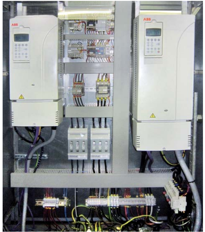
The compact ACS800-01 drives with built-in anti-sway control program installed in the cabinet.
