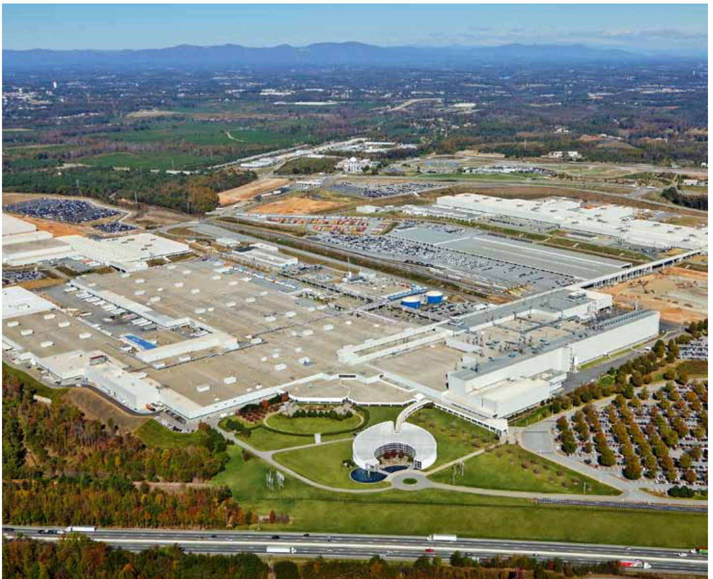
The BMW Spartanburg production plant in South Carolina.
