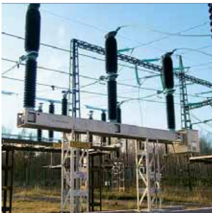
8 Live Tank Breaker D for voltage levels up to 170 kV and 40 kA breaking current.
