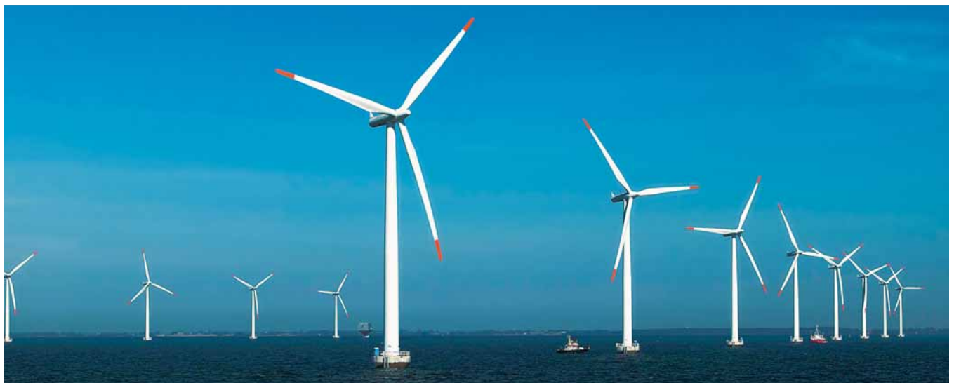
1 The Nysted wind park consists of 72 wind turbines, each with a max capacity of 2.3 MW
