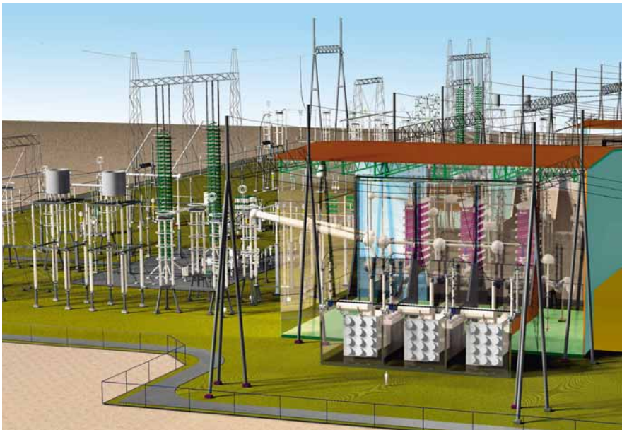
7 An HVDC converter station with four power blocks – the configuration is chosen to minimize the effects of individual component failures
