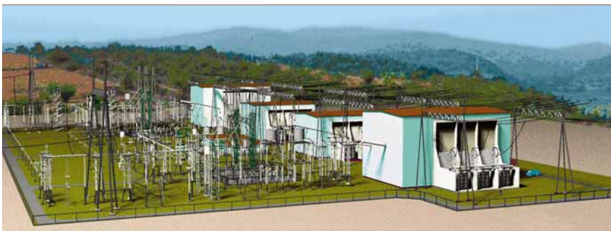
7 An HVDC converter station with four power blocks – the configuration is chosen to minimize the effects of individual component failures
