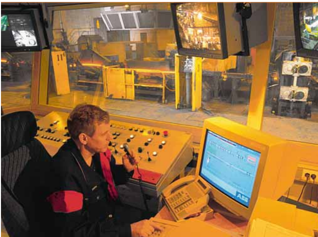
1 Operator's booth with control and monitoring equipment
