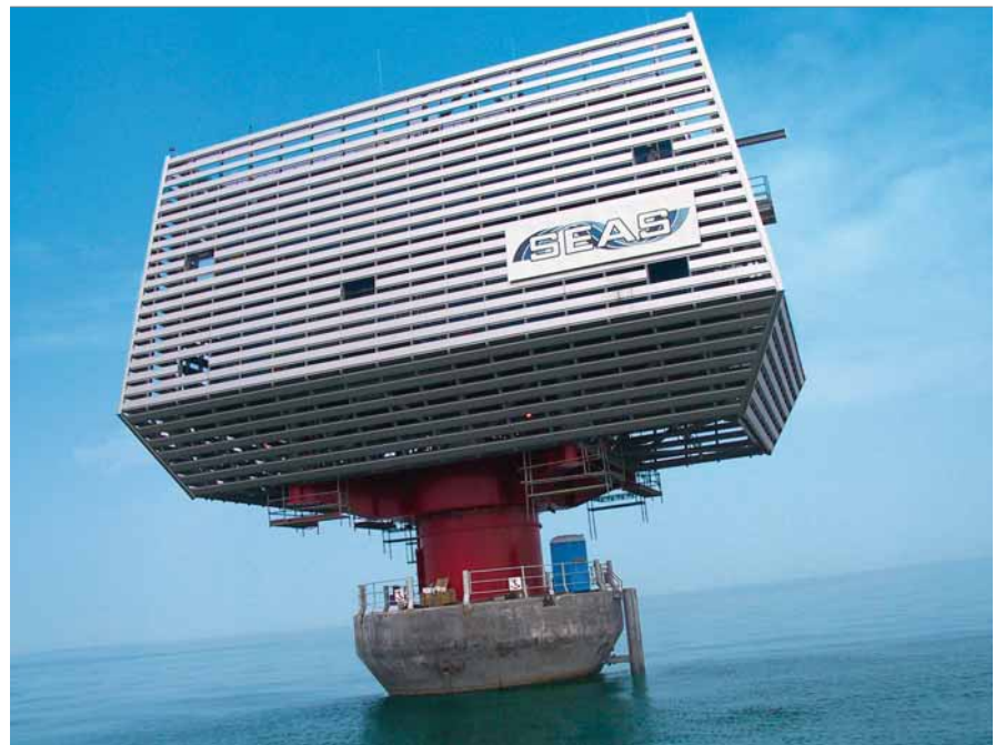
2 Transformer unit for the aggregation of the 72 wind turbines of the park
