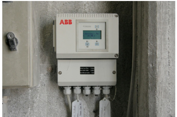
Fig. 3: The separate electronic controls for the CoriolisMaster MC2
