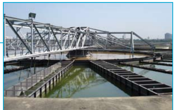
Clarifier at MWA's Bangkhen water treatment plant
