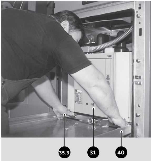
Figure 9/21: Withdrawal of the withdrawable part with circuit breaker onto the service truck. - Service truck engaged with the panel - Move the sliding handles inwards to disengage 31 Withdrawable part with VM1-T circuit breaker 35.3 Sliding handle 40 Service truck
