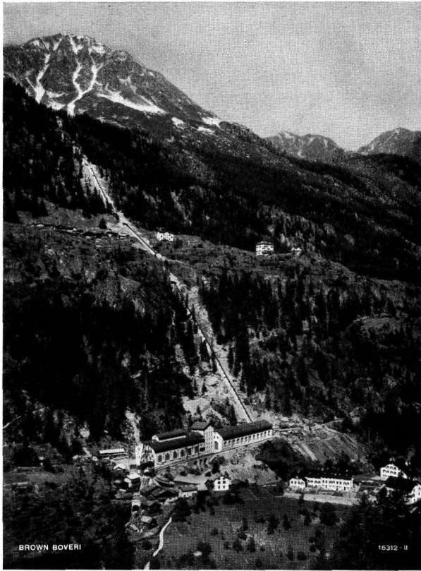
Fig. 5. — General view of the power station and pipeline.
