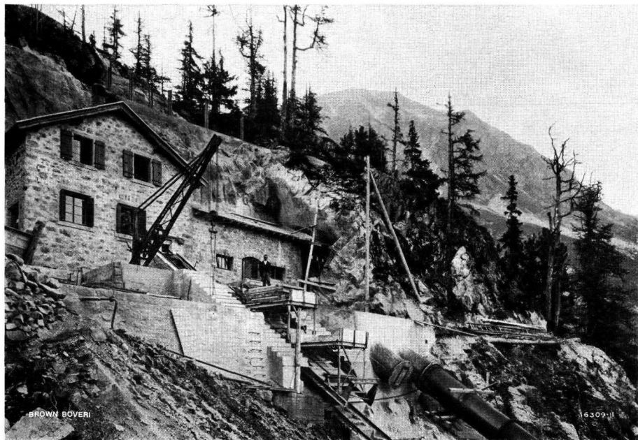
Fig. 2c. — Head of the pipeline during construction.
