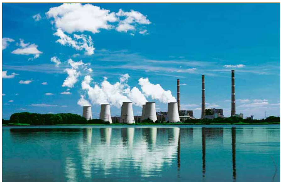
2 Typical application area for oxygen sensors: emission monitoring in power plants
