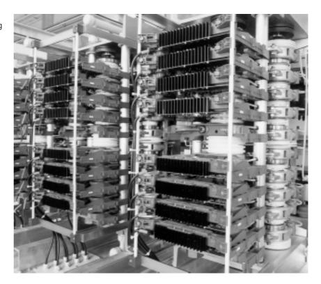
The two DVR systems are being used by an Israeli customer for microprocessor manufacture. These power quality systems are used to protect cost-intensive and sensitive manufacturing processes of the kind used, for example, in the semiconductor or papermaking industry. They compensate voltage fluctuations, so preventing production failures.
