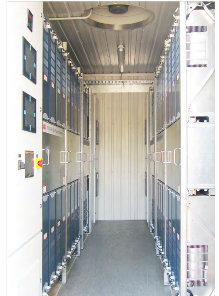
Two 1250 kVA PCS100 SFCs installed at Viktor Lenac shipyard
