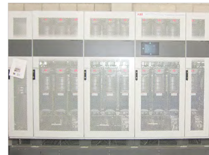
Providing grid interconnection from 50 Hz to 60 Hz
