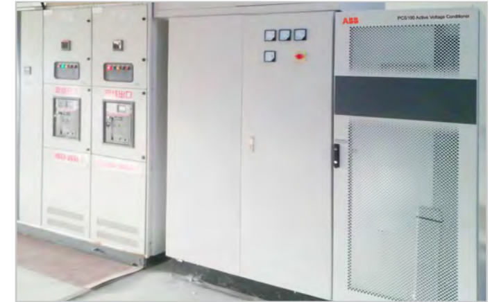
PCS100 AVCs are protecting two of the four transformers in the welding plant
