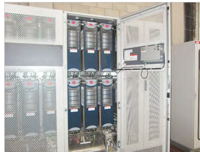
ABB's PCS100 1250 kVA Static Frequency Converter installed at Sinterama
