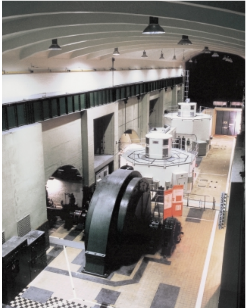
The two new generators in Porjus Hydropower Center. In the foreground, behind the older machine, is unit U8, which is used for maintenance training and studies. Behind it is the radically new Powerformer, which was commissioned in 1998 as U9.
