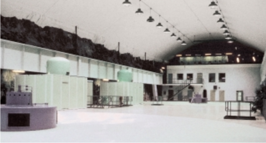
The New Projus hydropower station is one of the largest on the Lule river. The 267-MVA generating sets, with a diameter of more than 17 m and weighing 1,200 t each, rotate at a slow 83.3 rev/min. 2
