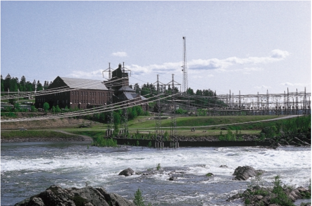
Porjus Hydropower Center is housed in an old hydroelectric power station in northern Sweden. The center was founded to provide facilities for R&D in the hydropower field and for training operative and maintenance staff under real-world conditions. (Photo: Kurt Westfeldt, Jokkmokk)
