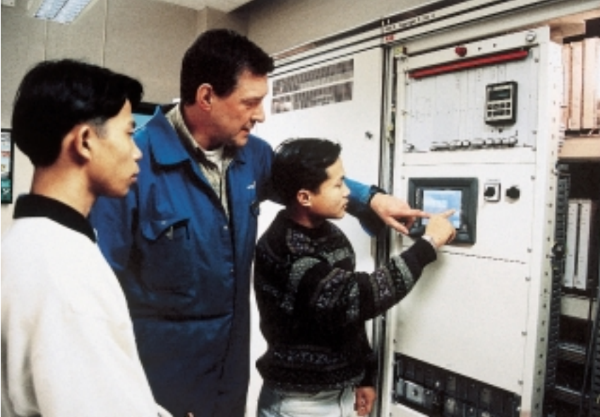
Certain operating information can be read directly off the control cubicles in the control room. Training is given by instructors from the Jokkmokk School, which can also access all the operator functions at the center via modems. 8
