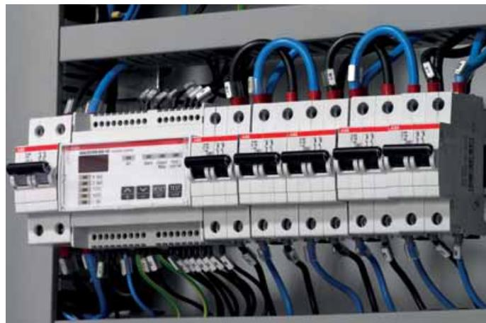
This is an insulation monitoring device for group 2 medical locations fully compliant with the IEC 60364-7-710 reference standard. It integrates all the performances established by the reference standard, such as overload and overcurrent monitoring, together with traditional IT system earthing insulation measurement.
