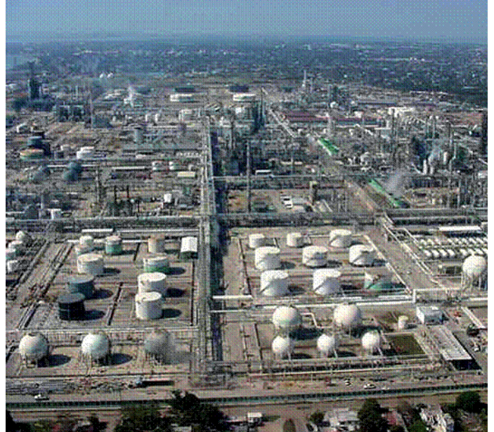
View of PEMEX's Madero refinery
