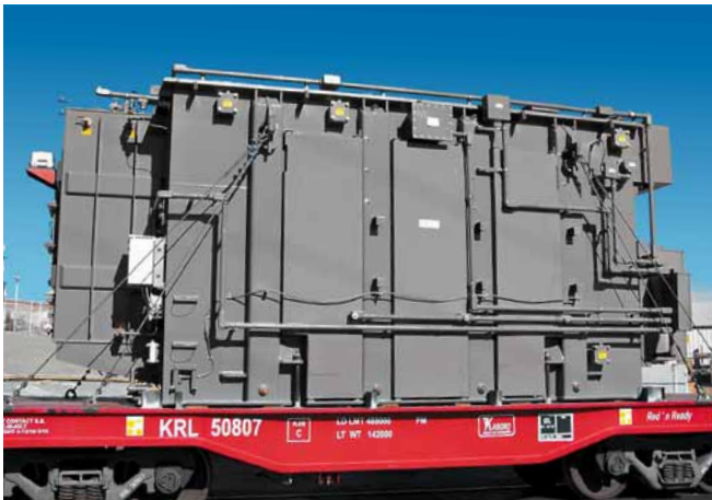
10 Ultra-low noise ConEd transformer with Sound Panels
