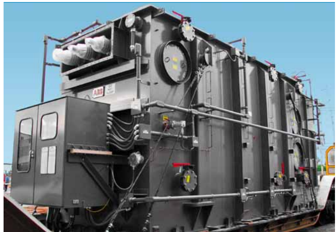
11 Ultra-low noise ConEd transformer with no Sound Enclosure or Panels
