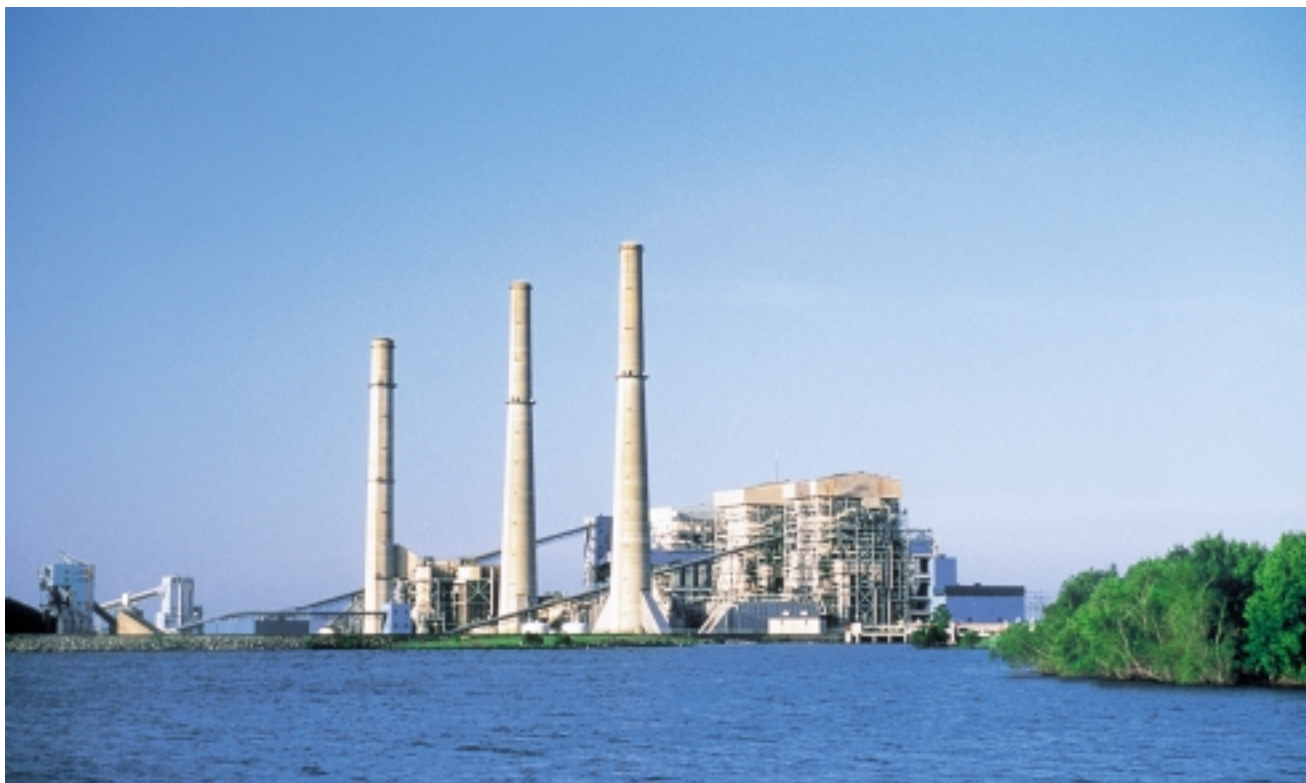
Fayette power plant of the Lower Colorado River Authority, in La Grange, Texas. The coal-fired plant has 3 boilers with nominal ratings of 600/600/450 MW. All three are equipped with ABB electrostatic precipitators.
