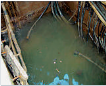
Two SDTs have been operating under salt water at the Charleston Historical Center in South Carolina since May 2000.
