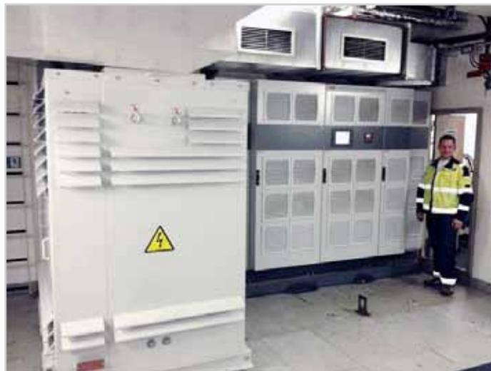
ABB's PCS100 Static Frequency Converter
