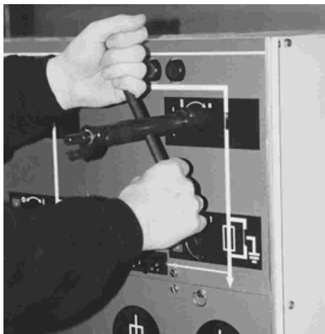
Earthing switch: Close: Turn the operating handle clockwise. Open: Turn the operating handle anti-clockwise.
