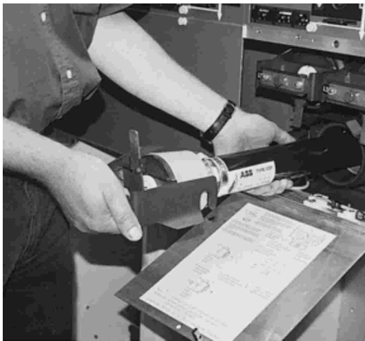
6. Pull out the fuse handle. The fuses are firmly fixed in the fuse cover.
