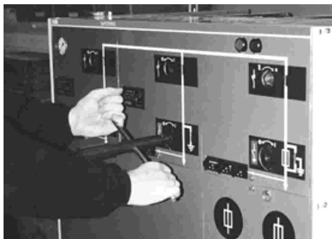
Earthing switch: Close: Turn the operating handle clockwise. Open: Turn the operating handle anti-clockwise.
