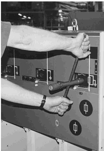
2. Close earthing switch by turning operating handle clockwise.
