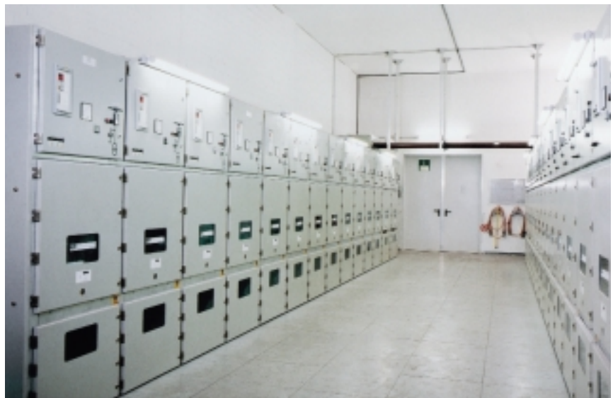
The new medium-voltage switchgear of type ZS1. The installed withdrawable vacuum circuit-breakers are also suitable for motor-switching.
