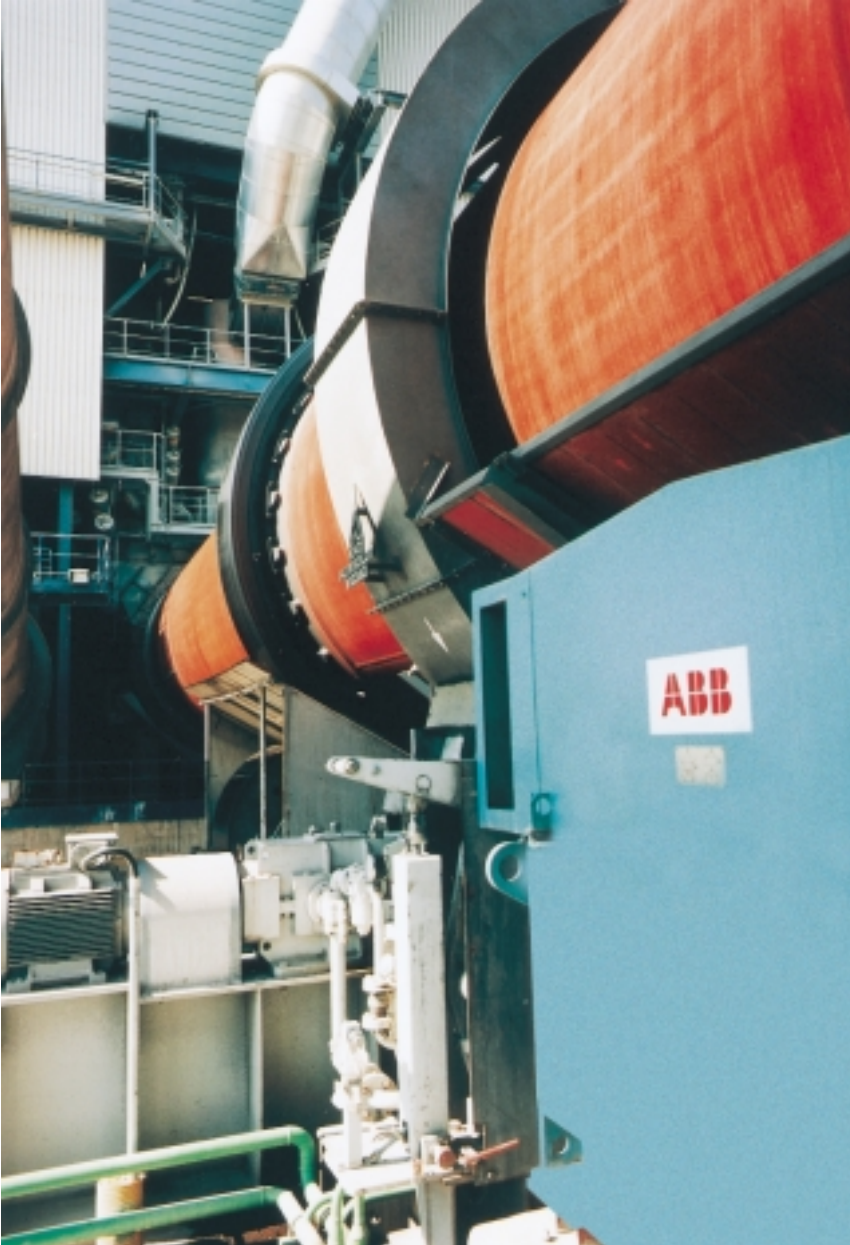
The rotary kiln is driven by two frequency converter drives with 490-kW motors.
