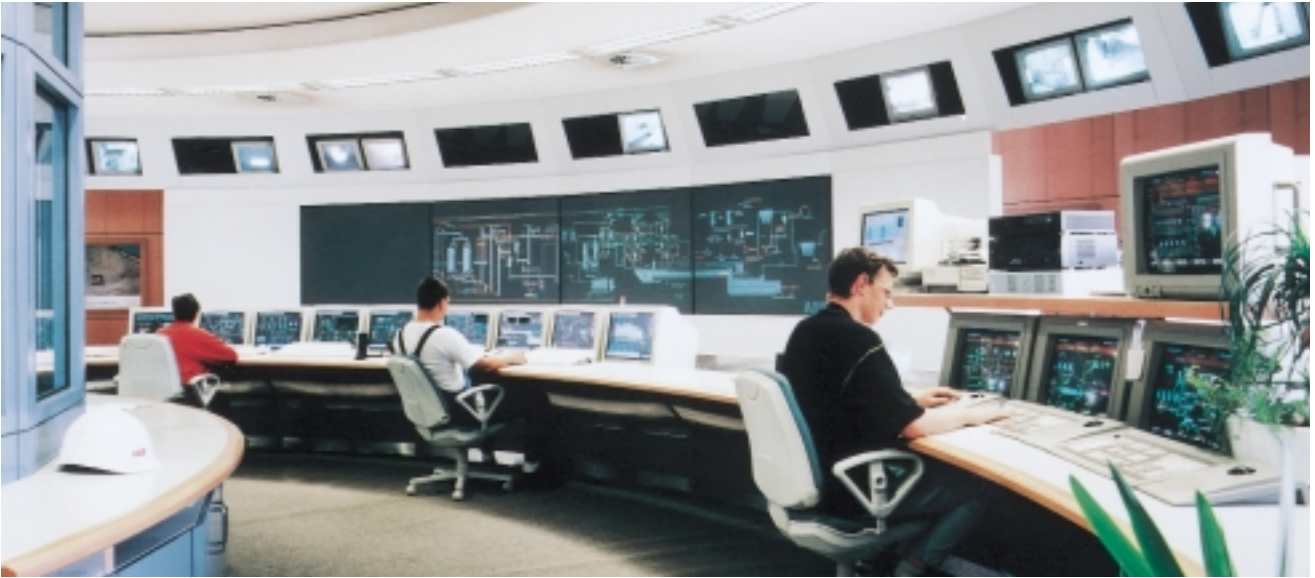
The new central control room. Located next to the new kiln line 5, it replaces 12 decentralized control rooms.
