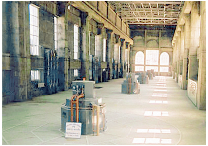
The canal head power house of the Sardar Sarovar dam with the five Kaplan turbines.
