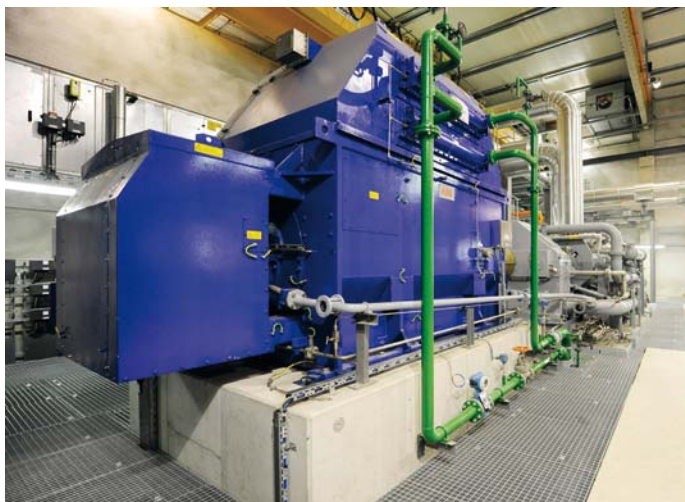
15.5 MW 4-pole ABB motor powering one of the compressors (source: RAG/Steve Haider)
