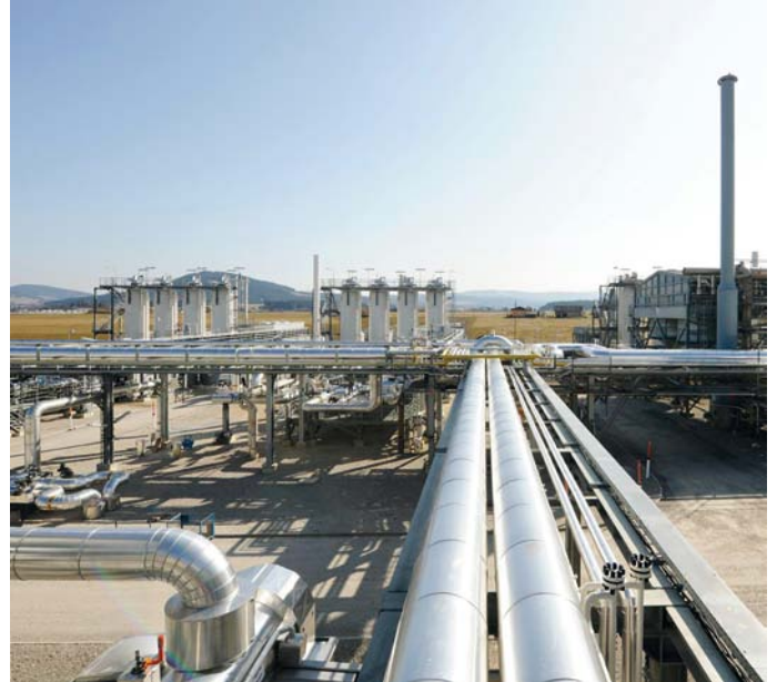
Haidach underground gas storage facility in Austria (source: RAG/Steve Haider)
