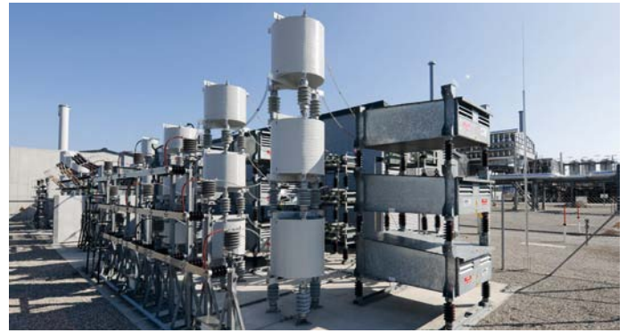
Harmonic filter and power factor compensation equipment (source: RAG/Steve Haider)
