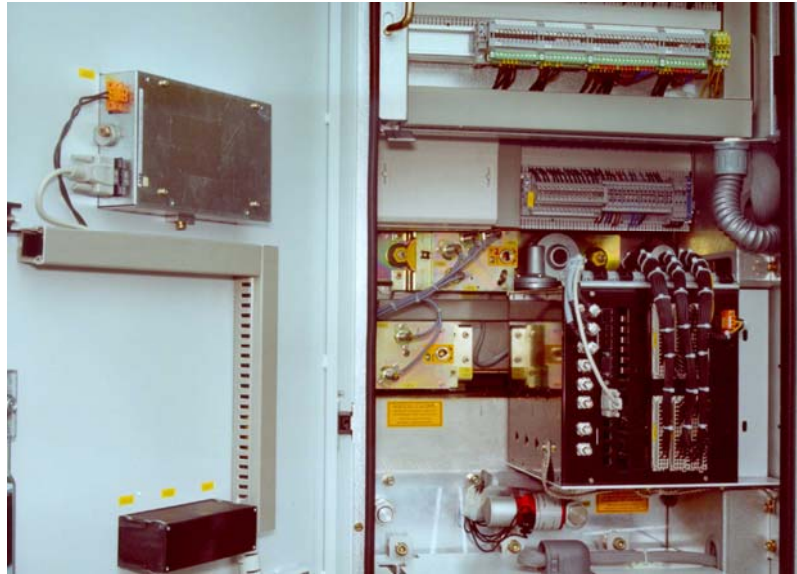
Figure 20: Example of mounting of the Central Unit in the LV compartment and the HMI on the door
