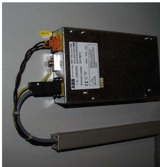
Figure 23: Grounding of the REF542plus HMI Local Control Unit
