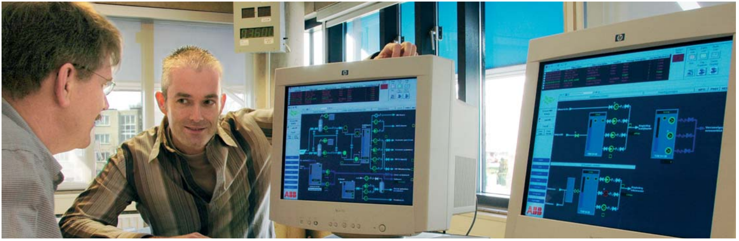
Mr. Ing Remko van Duin, process coordinator at WSHD Dokhaven, with the Process Portal operator stations in the control room. Van Duin is satisfied with ABB's work.
