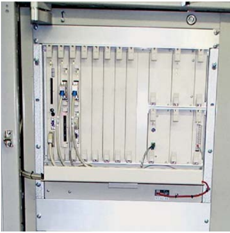
Since the old controllers had reached the limits of their capacity, new ones had to be installed.
