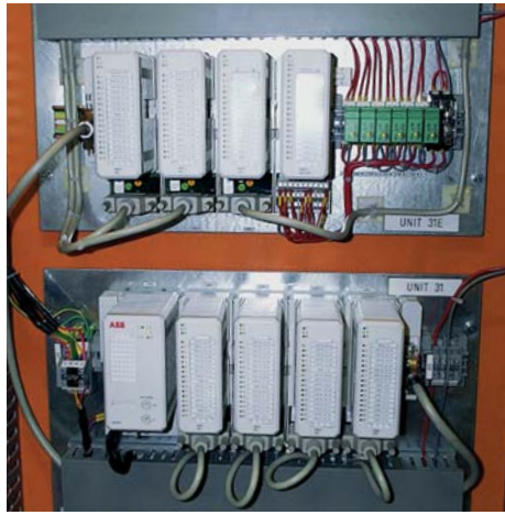
The I/O units of the old MasterPiece 100 controller were replaced with the S800 I/O.
