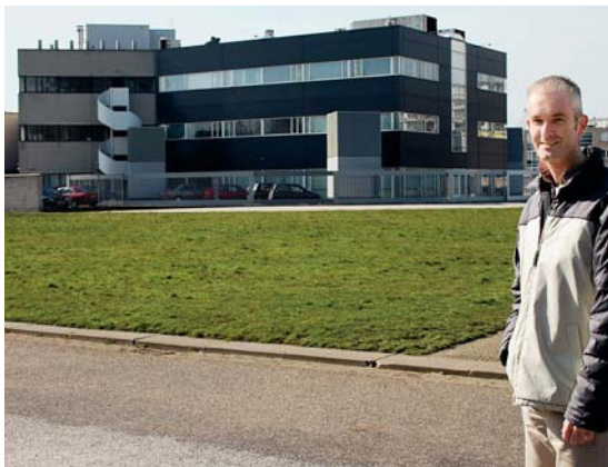
The Dokhaven facility, an underground water treatment plant in the middle of Rotterdam, is built in a former harbor. The water is treated at a pump station situated 14 meters under the river; during this unique process, it pumps up the treated water so that it flows to the river.
