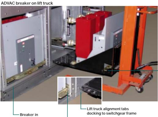
Tabs secure breaker to lift device for safe handling
