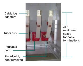
Cable Compartment (Main bus cover installed)
