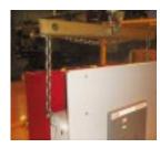
An optional lifting yoke is a simple hook, chain and spreader bar assembly used to lift circuit breakers with an overhead crane or hoist.
