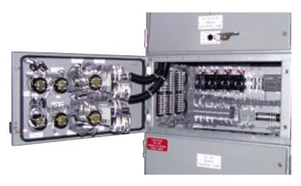
Modern microprocessor technology enables consolidation of multiple protective and instrumentation functions for all phases into fewer devices. Therefore, most relays and controls can be mounted on isolated low voltage compartment doors. In some cases, the use of discrete relays or extensive protection systems dictate mounting instruments on primary compartment doors. In these situations, 10-inch front frame extensions provide adequate depth for virtually all door-mounted instruments. These frame
