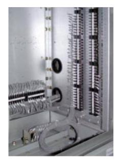
38-inch instrument compartment with TOC switch and terminal blocks for customer wiring and interframe connections.
