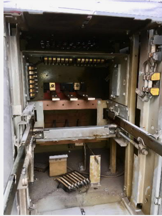
AKD-5, AK 25 Cassette or Substructure, Rails Extended
