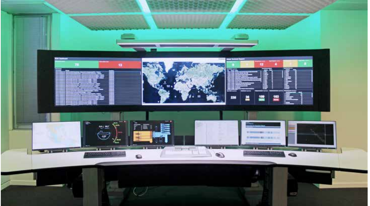
ABB's Integrated Operations center takes ship support to the next level
