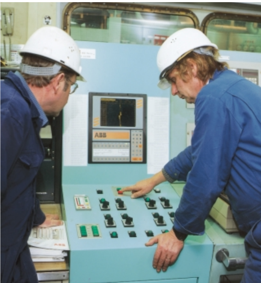
Addition to the control desk for operating the booster system
