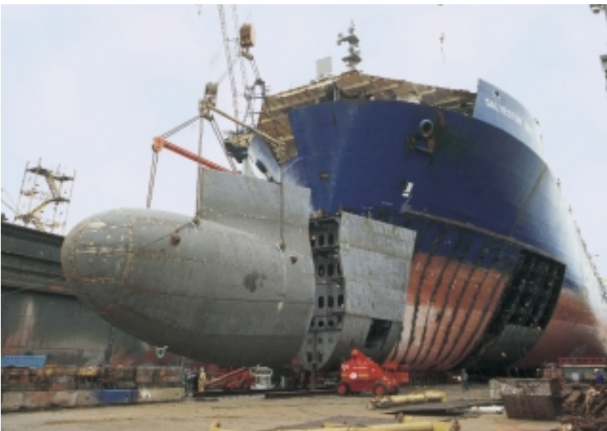
The new forebody is brought into position. 3
