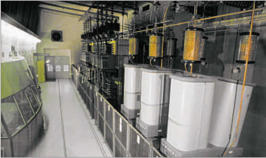
Gotland 1 extension, with the world's first HVDC thyristor valves
