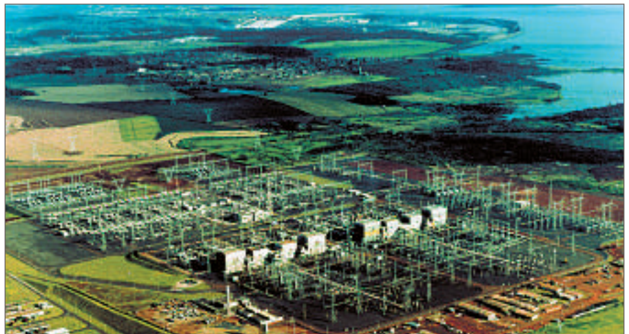
Foz do Iguaçu converter station with the Itaipu 12,600-MW power station in the background
