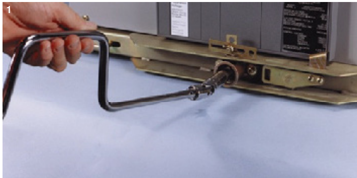
1 Racking crank | 2 AMVAC manual opening handle | 3 Lift truck | 4 Test jumper | 5 Test cabinet
