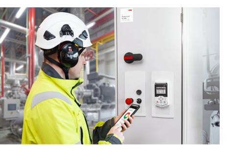
ACS800 single drive modernization is a fast, flexible, and environmentfriendly solution to extend the equipment's lifetime. The service modernizes the existing ACS800-07, -17 or -37 drive with state-ofthe-art ACS880 technology without the need to fully replace the drive cabinet. This optimizes costs and minimizes the downtime of your operations.
