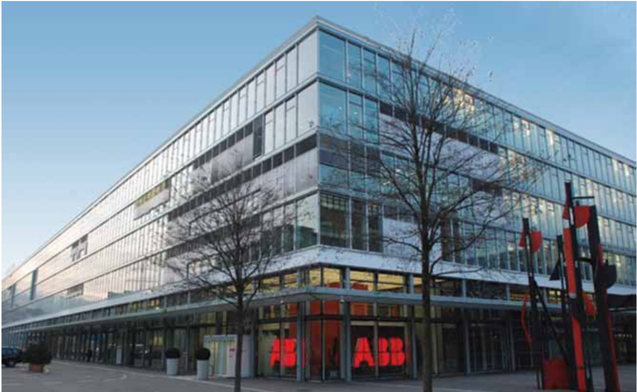
ABB's headquarters in Zürich
