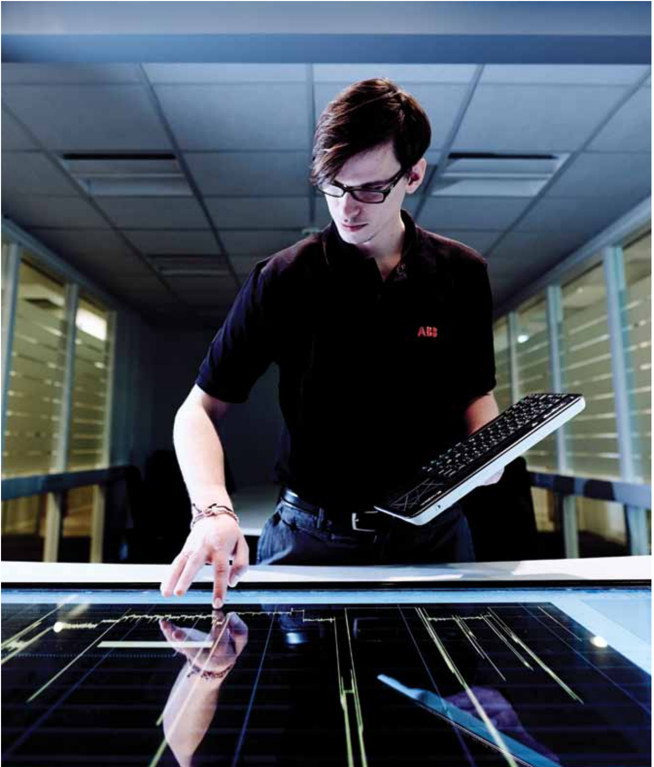
Integrated Operations Center at Billingstad
