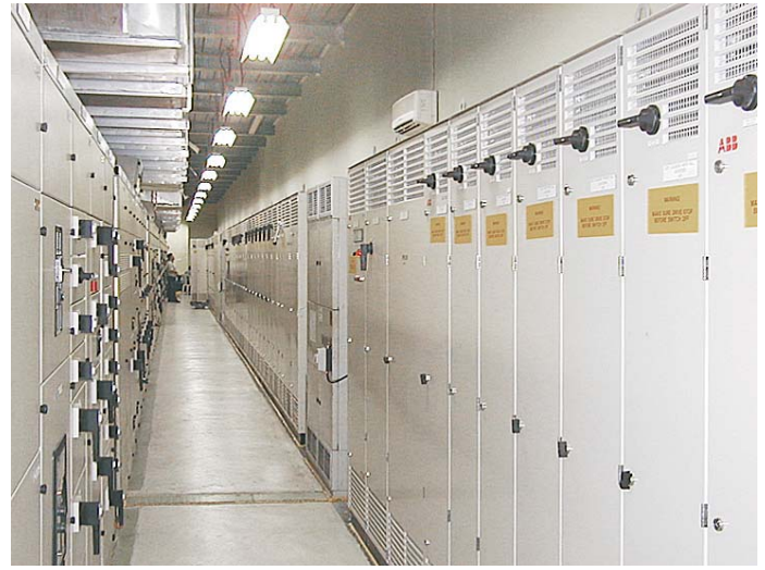
ACV700 drive cabinets
