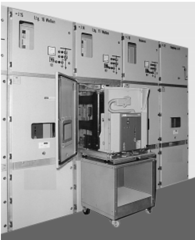
Figure 3/10: Service truck with withdrawable part in front of the open circuit-breaker compartment in a switchgear
