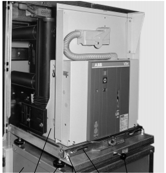
Figure 6/10: Withdrawable part standing on service truck and secured in the catches
