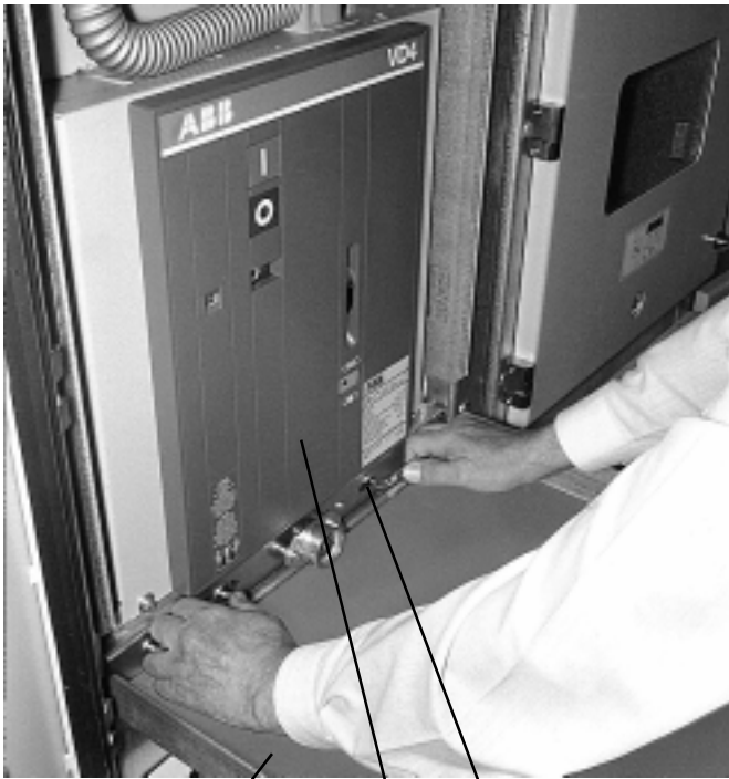
Figure 6/9: Service truck engaged with the switchgear panel. Withdrawable part released for withdrawal with the handles slid inwards.
