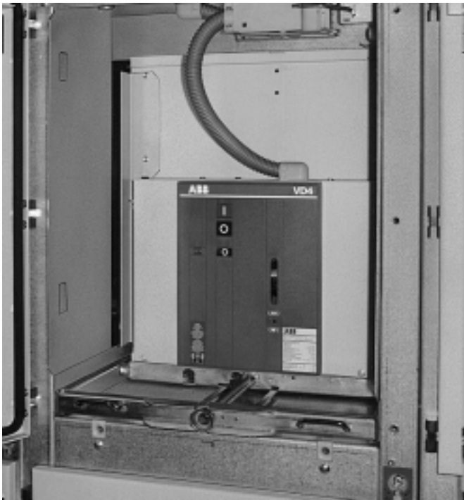
Figure 3/6: Circuit-breaker compartment, opened. Withdrawable part in service position.
