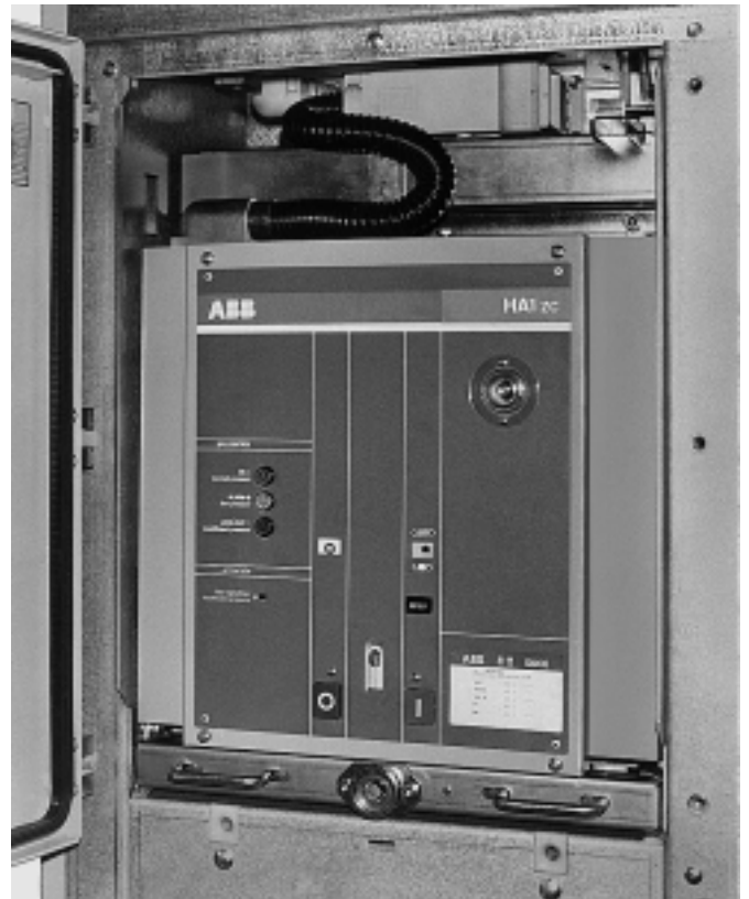
Figure 3/17: Withdrawable part with circuit-breaker, type HA, shown in test/disconnected position
