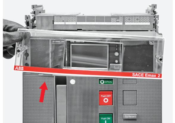
**3** Manually remove the racking in and out lever located in the bottom part of the circuit breaker.
