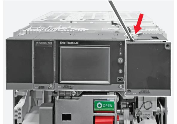
**35** By means of the cutter start removing the label located on the Ekip measuring blind module and by means of the pliers complete the removal operation.
