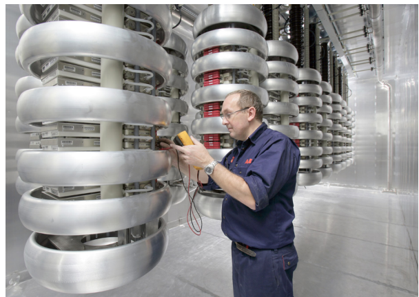
An ABB engineer tests HVDC Light valves during installation
