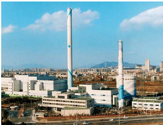
Gangnam is a combined heating and power plant in Seoul, the second largest plant of KDHC, supplying 134 000 households with district heating. The demand is ever increasing.
