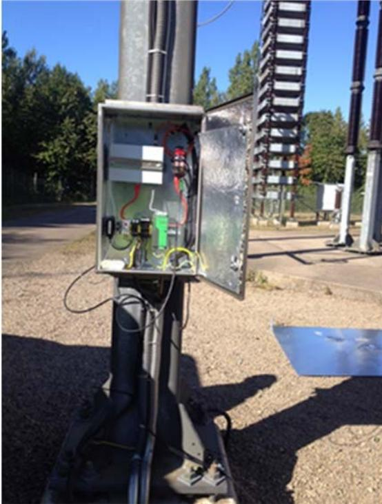
**Figure 4 Junction box with current monitor and detector unit installed in Baltic Cable**
