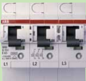
Protecting the locked position with a cable tie
