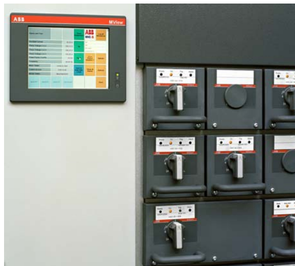
Figure 15 MView in MNS iS Switchboard
