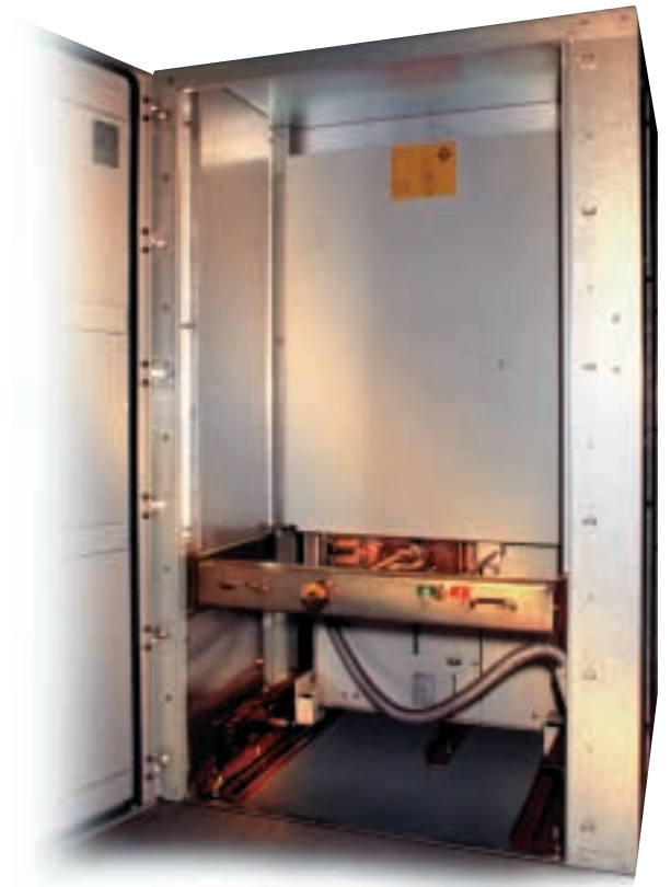
Opened circuit-breaker compartment, withdrawable part in service position
